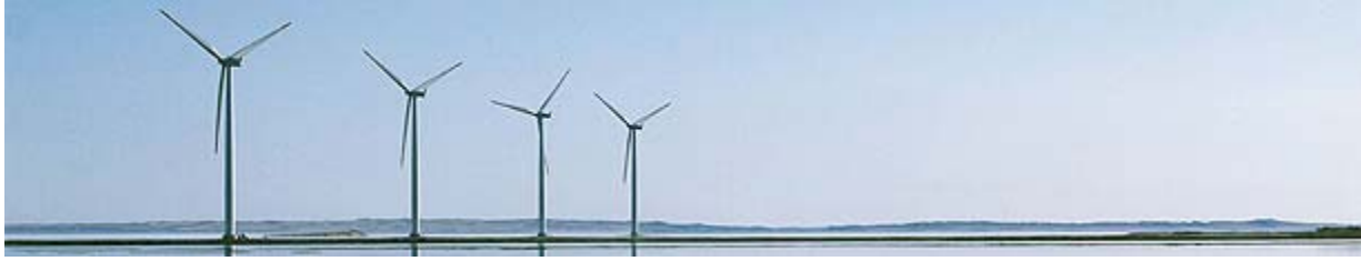
Figure 4. Siemens 2.3 MW Turbines
