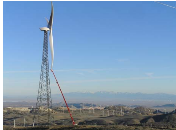
Figure 31. Knight & Carver Swept Blade Mold and Flight Testing
